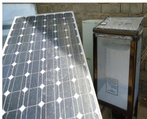
Fig. 3, solar electricrefrigeration system
